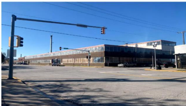
Looking south-west from the corner of Swift St. & E. 16 th Ave.
